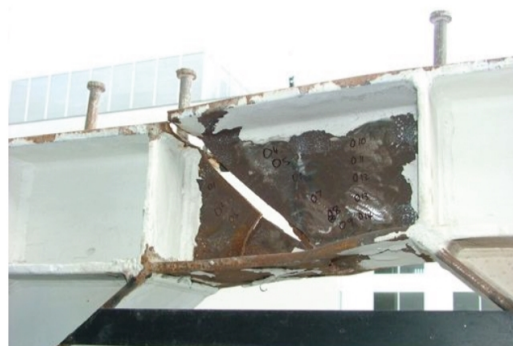
Figure 2. EBF link after removing from its location. (Ferguson et al., 2013)
