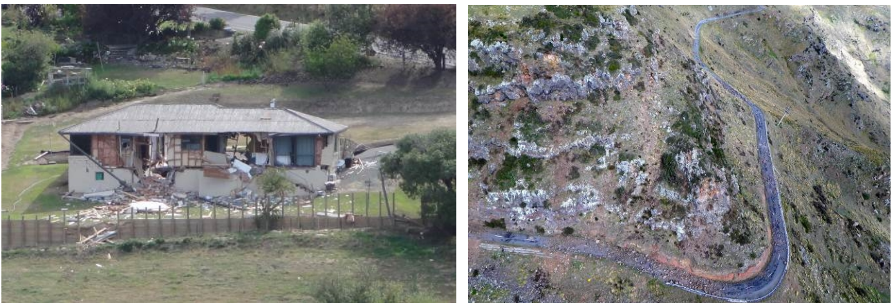
Figure 7: Rockfall damage to houses and roads
