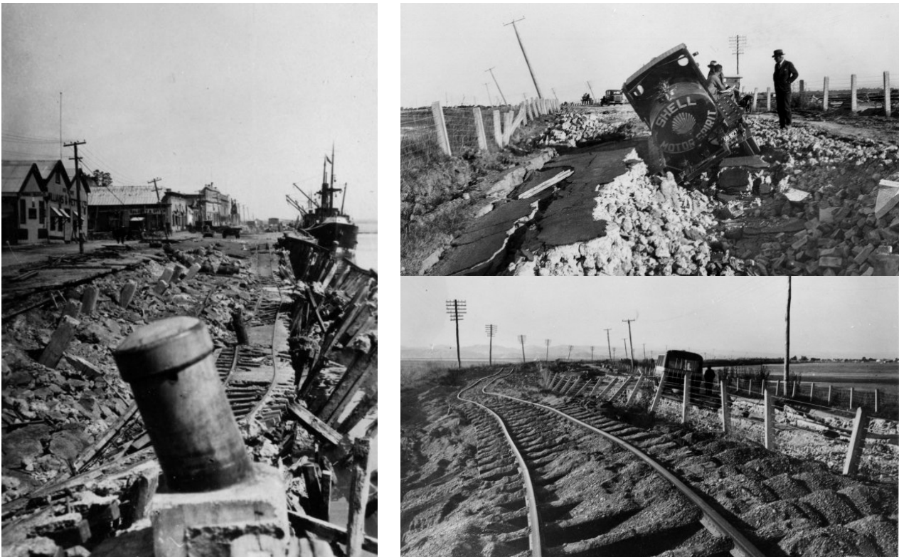
Figure 3: Damage to infrastructure from geotechnical failures in the 1931 Napier earthquake
