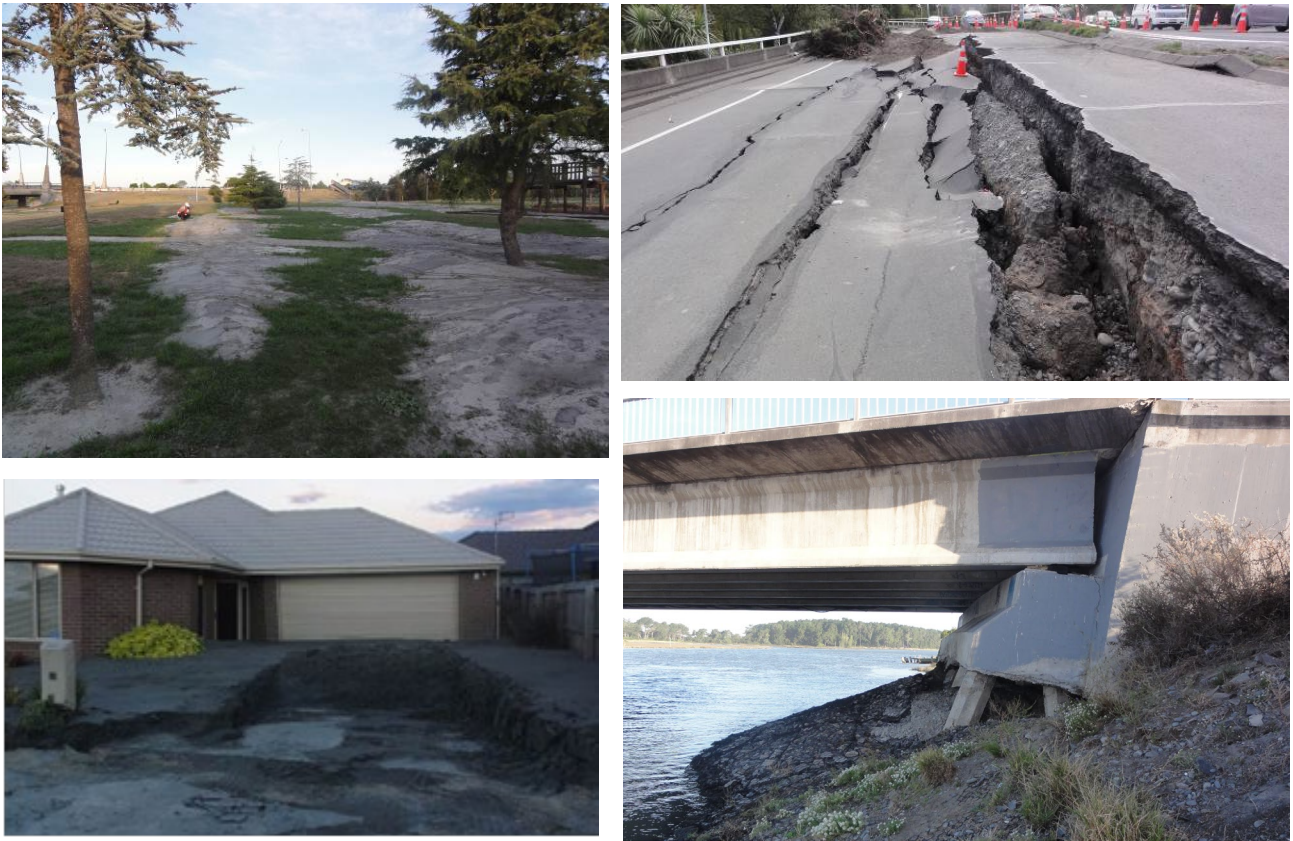
Figure 6: Liquefaction sand boils, ejection of sand and silt, and lateral spreading damage to transport
