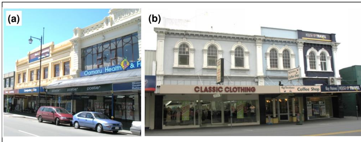
Figure 2. Examples of two-storey row masonry buildings with large openings along shopfronts from (a) Oamaru and (b) Ashburton. Reproduced with permission from Russell (2010).
