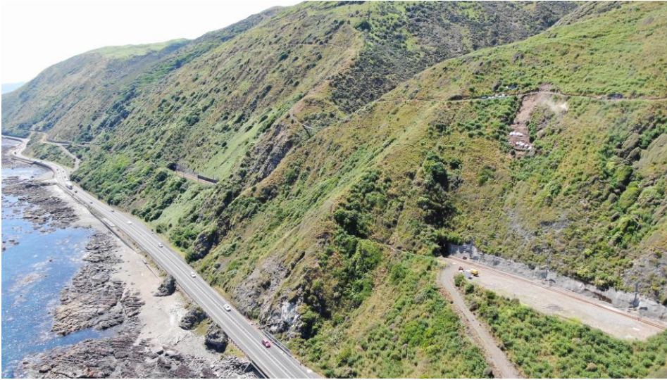
Figure 3: Paekakariki Escarpment – with multiple slope hazards affecting road, rail and the Te Araroa (TA) trail. Works to mitigate NIMT 33.44 slip site visible at upper right
