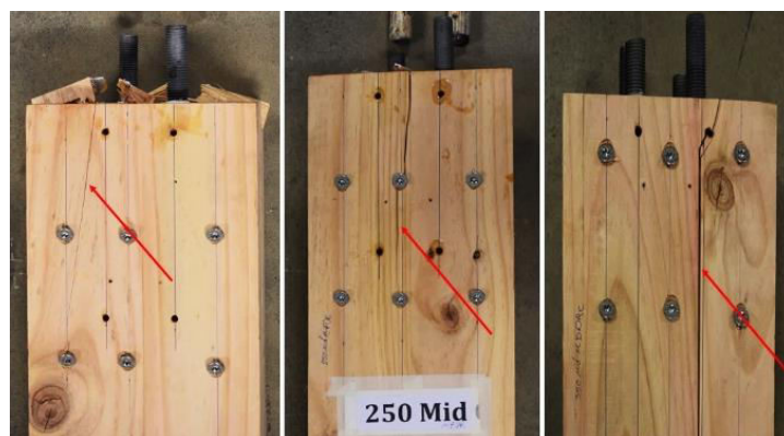
Figure 7. Surface crack of specimens containing rods on the boundary of two cross-wised layers.
