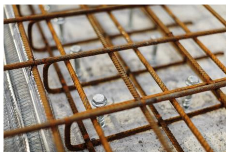
Figure 1: Concrete overlay application using post-installed mechanical anchor
